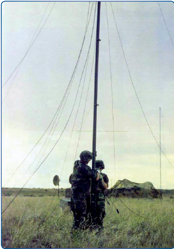
These tough, composite push-up masts can be erected by a two-person team in under 10 minutes.
